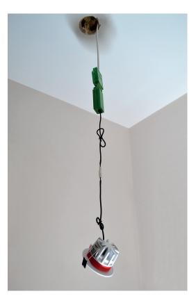
**4.** Once the downlight has been removed from the ceiling, the driver will be the next out. When you have this out, you will then need to disconnect it from the downlight (fig. 9, 10).
