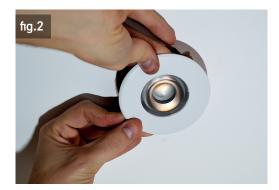
**3.** As you pull the downlighter from the ceiling, **you must hold on to the spring loaded retaining clips** to avoid them springing back and trapping your fingers or damaging the plaster board as shown in fig. 4. Once the springs and fitting are clear from the ceiling, they can then be released gently back to their unloaded position (fig. 8).
